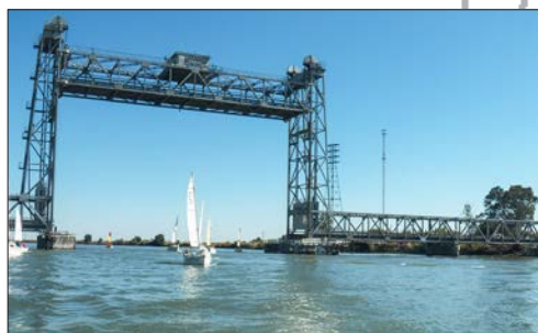
Three Mile Slough Bridge
