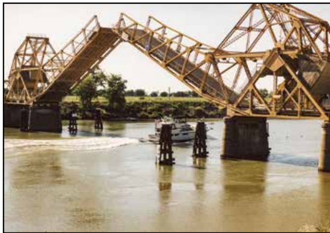
The Paintersville Bridge. Photo: Jan Vick
